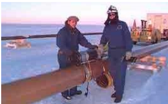
Radiography of weld joints.
