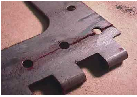
Indication of cracks running between attachment holes in a hinge
